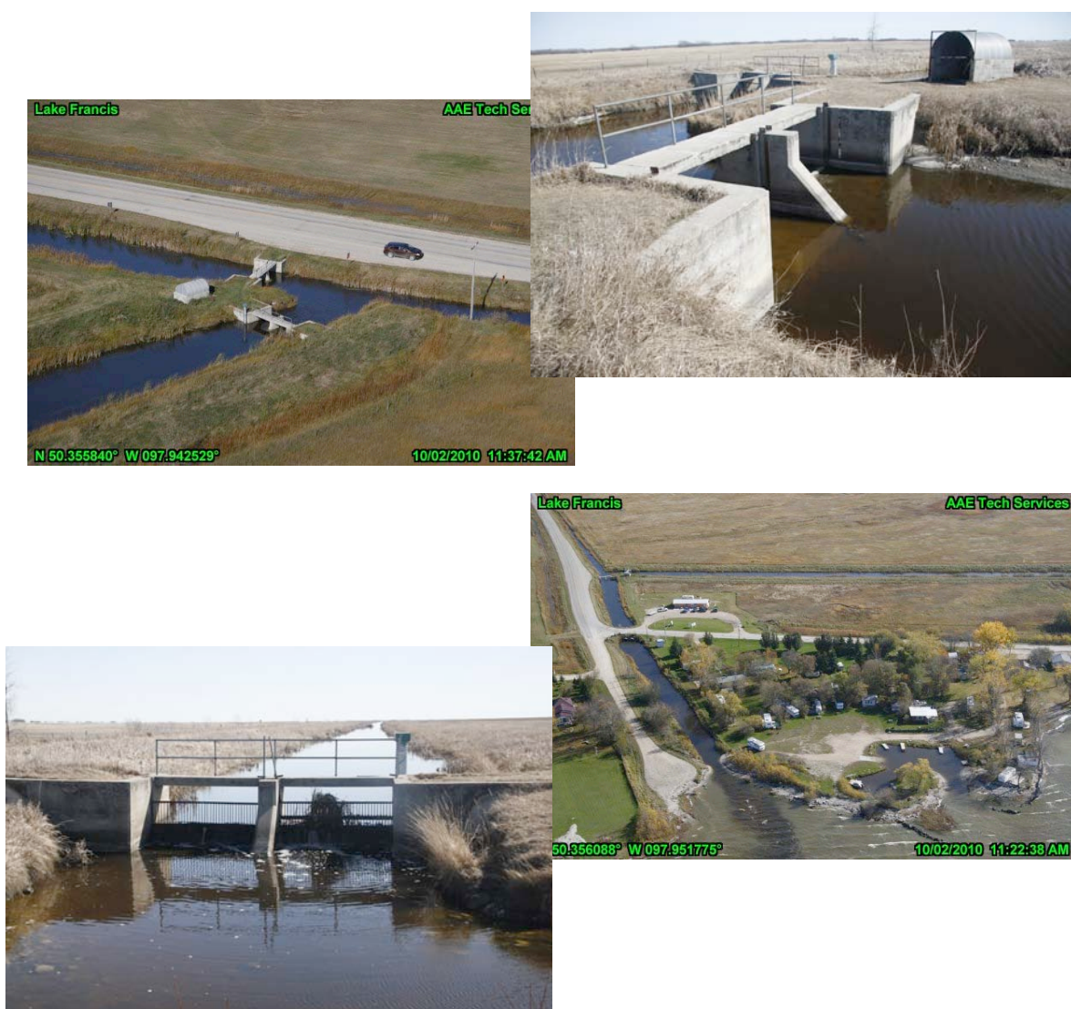
Figure 6. Photographs of the screened control structure within the outlet channel of the Lake Francis.
